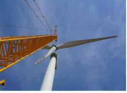
▲ Field replacement of 4-point contact pitch bearings by T-SOLID
