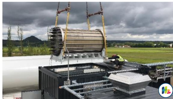
Stack under erection (outdoor case)
