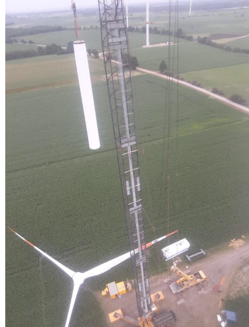
Demontage Vestas V80-100m NH
