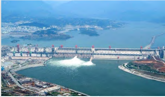
Connecting remote generation
