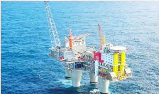
Power from shore / Ship to Shore
