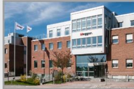
Facility Danderyd (Sweden)
