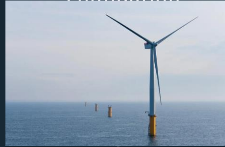
Transition Piece and Foundation
