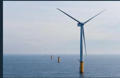
Transition Piece and Foundation
