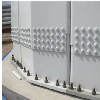
Foot flange and lowest friction joint connection of the BSS towers (Siemens Wind Power, 2012).
