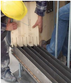
Perforated plate connection ( http://bit.ly/1M79bbW ).
