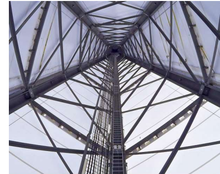
Interior view of the space frame tower (GE, 2014).
