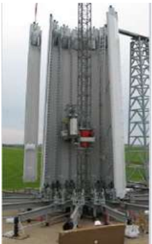
Assembly of a segment of the BSS Towers (Siemens Wind Power, 2012).
