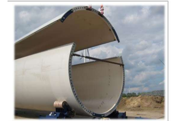
Assembly of the LDS towers (Nowack, 2014).
