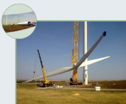
CONSTRUCTION SUPERVISION & COMMISSIONING
